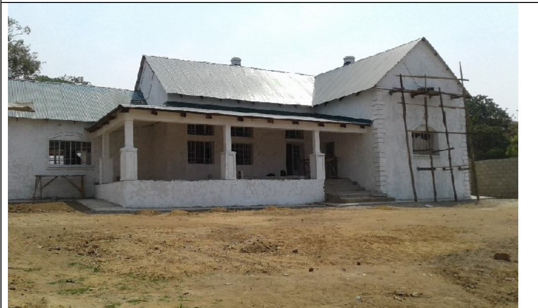
Refurbishment of the Blantyre District Registration Office (DRO) in progress
